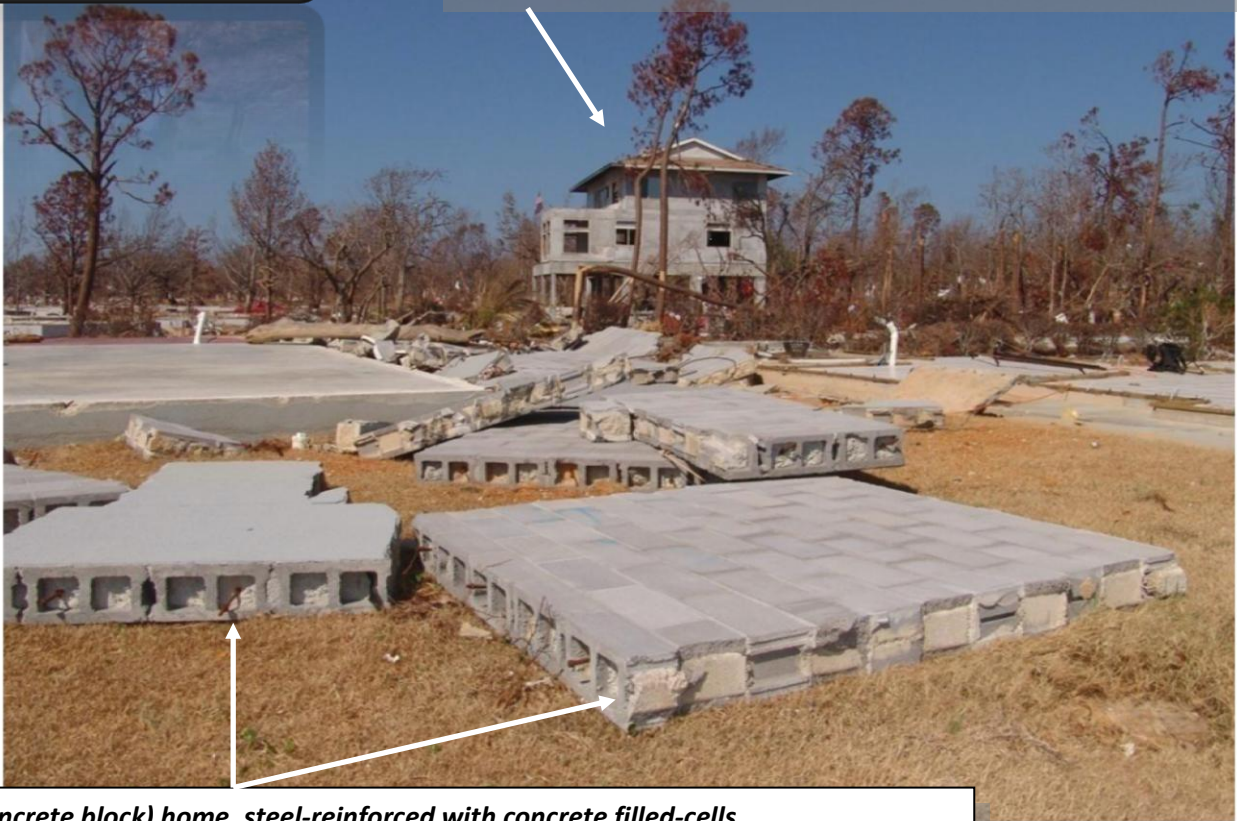
CMU (Concrete block) home, steel-reinforced with concrete filled-cells...
